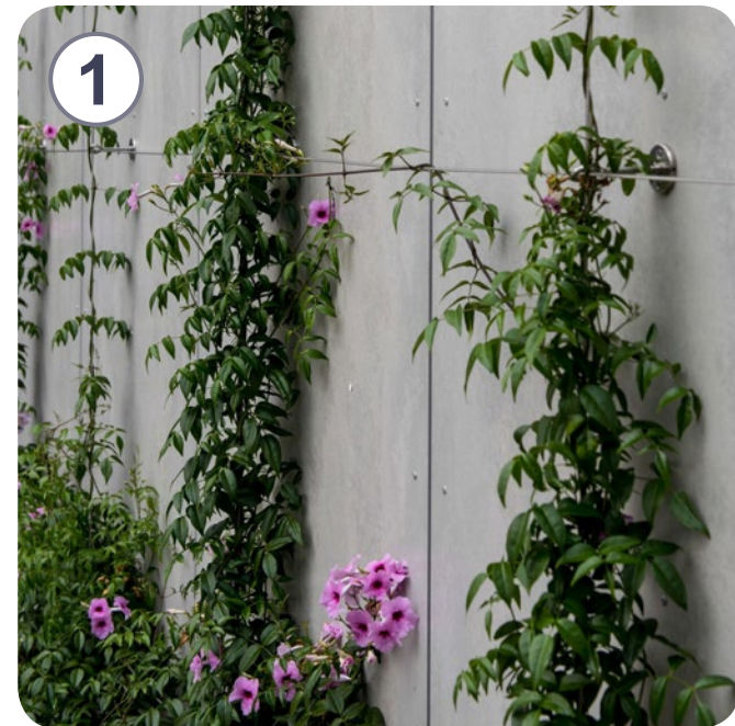
Flowering vines on screen structure
