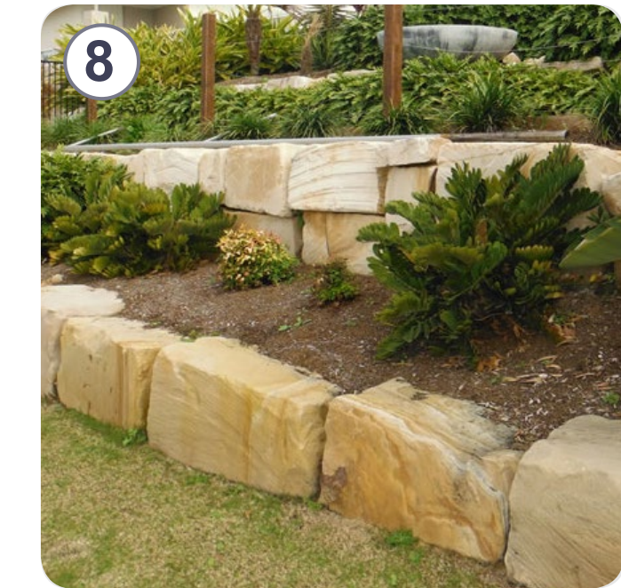
Sandstone seating walls
