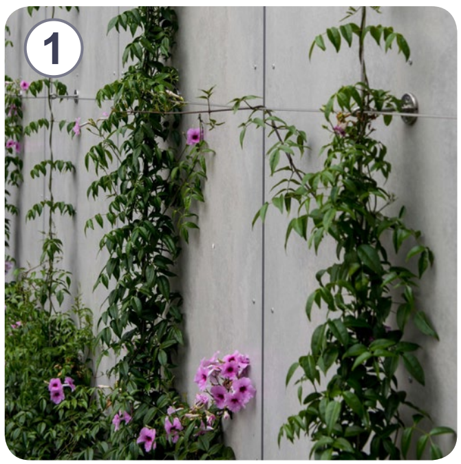
Flowering vines on screen structure
